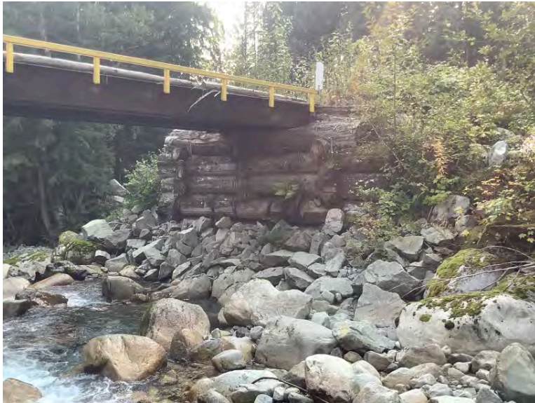
Right Bank Abutment when facing downstream
