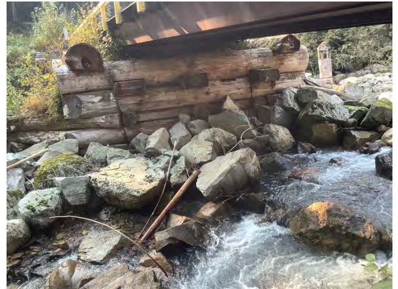
Midspan cribbing viewing from left bank
