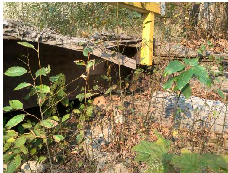
Left bank single sill bearing
