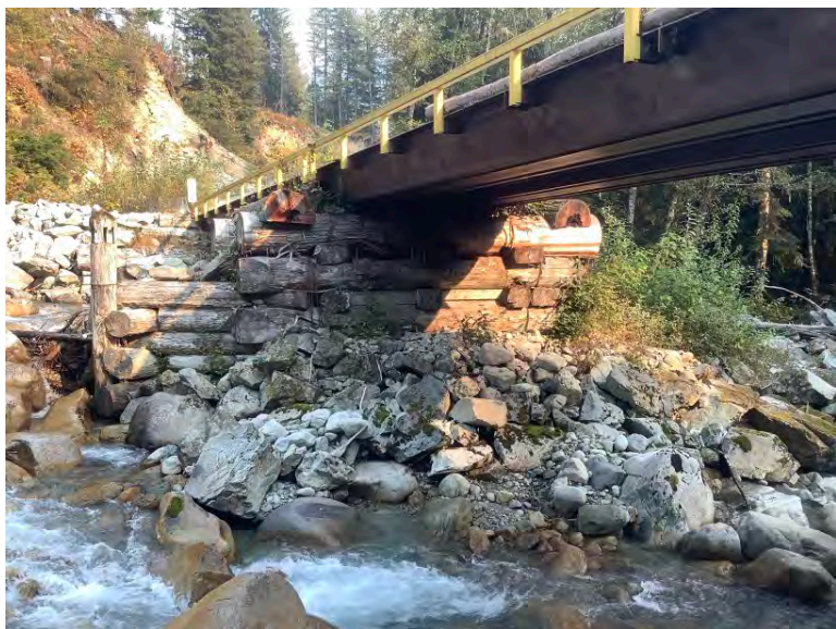
Midspan cribbing viewing from right bank
