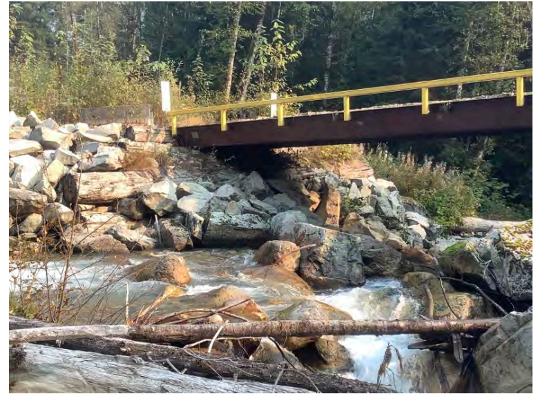
Left Bank Abutment when facing downstream
